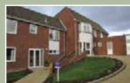
HEFFLE COURT HEATHFIELD
